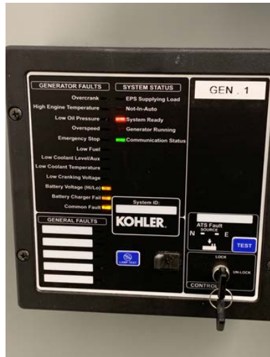
Working with GC and County on Generator Provisioning and Management
