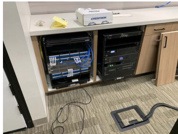
GC and County working on final solution and finish
